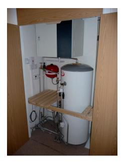
Good practice: MVHR unit (above cylinder) in easily accessible position and within the heated envelope of the home
