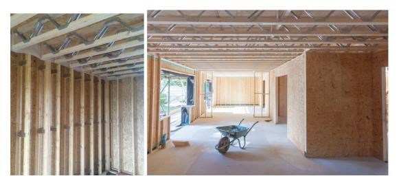
Twin-Stud Roof Structure, 400mm, Cold Bridge free, 0.102W/m2.K U-Value.
